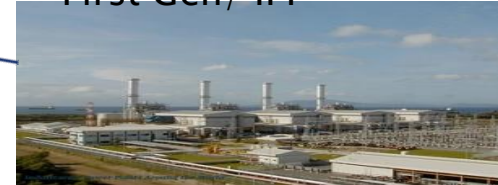
1,000 MW Sta. Rita First Gen/ IPP
