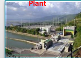
755MW CBK Hydroelectric Power Plant
