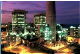
1294 MW Sual Coal-fired Power Plant
