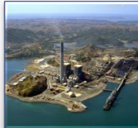
600 MW Pagbilao Coal-fired Power Plant
