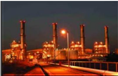
1060 MW Sta Rita Natural Gas-fired Plant
