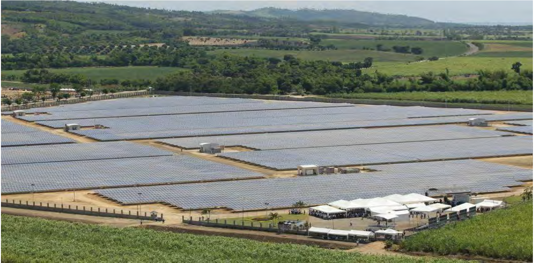
22 MW San Carlos Solar Project
