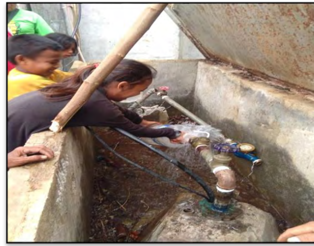
Energization of Evacuation Centers and Water System
