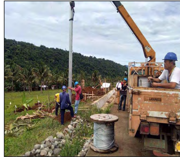
Erection of Poles by LASURECO Technical Staff at the Tent City
