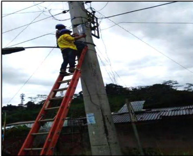
Installation of Street Lights
