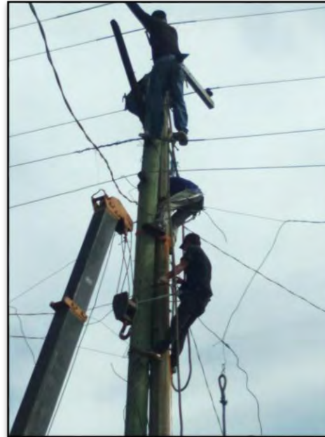
Replacement of Rotten Poles in Malabang, Lanao Del Sur
