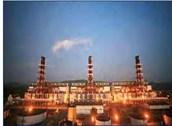
235 MW 1590ec Bauang Diesel Power Plant (La Union)
