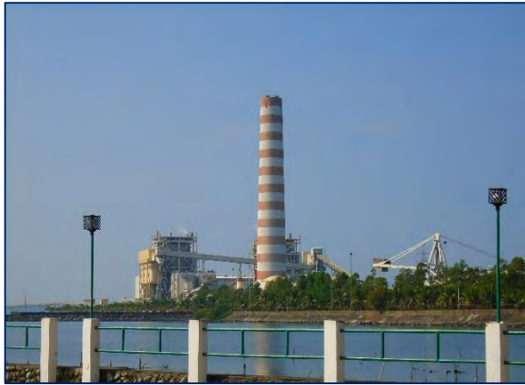
2 x 315 MW AES Masinloc Coal-Fired Power Plant (Zambales)
