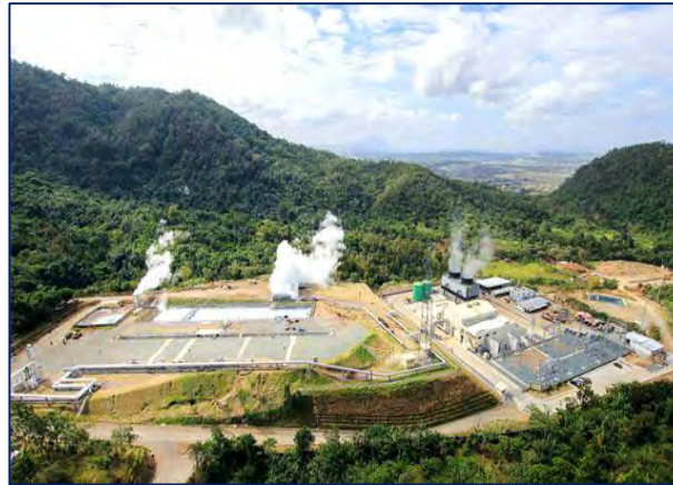
20 MW Maibarara Geothermal Power Plant (Batangas)
