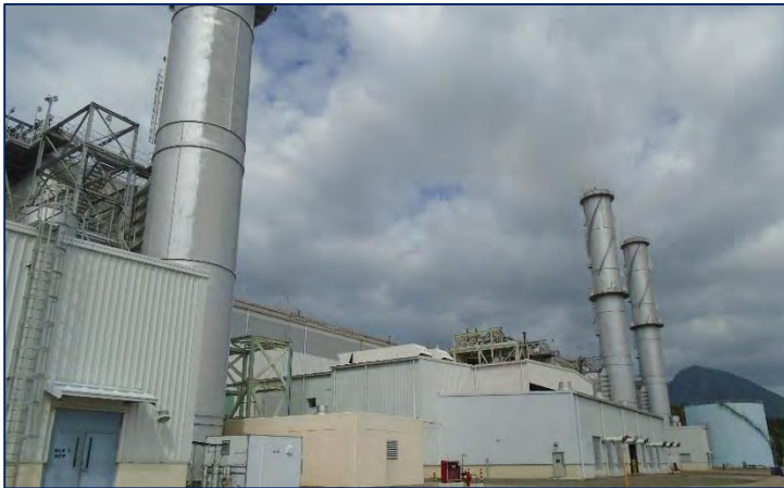
2 x 600 MW KEILCO Ilijan Natural Gas-fired Power Plant (Batangas)
