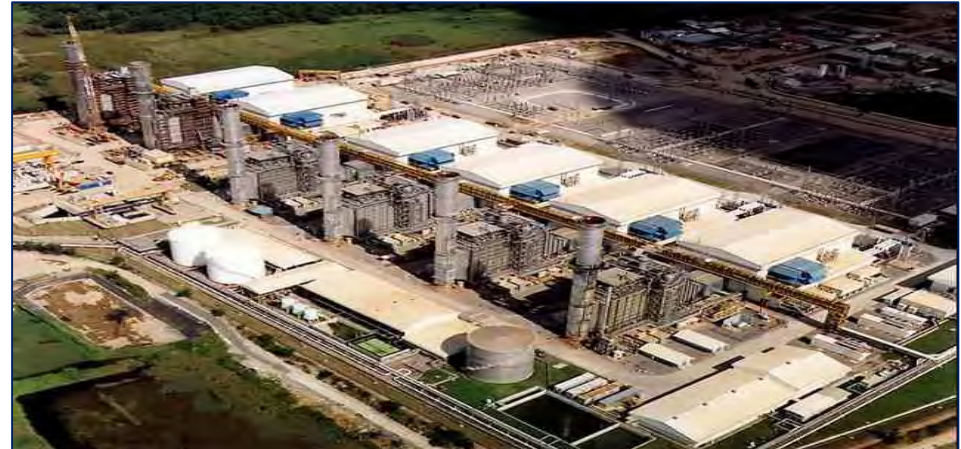
First Gas Power Corp. 2 x 250 MW San Lorenzo and 4 x 250 MW Sta. Rita Natural Gas-fired Power Plant (Batangas)
