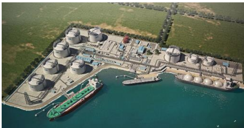
Figure 14: Singapore LNG with extra tanks for trading
