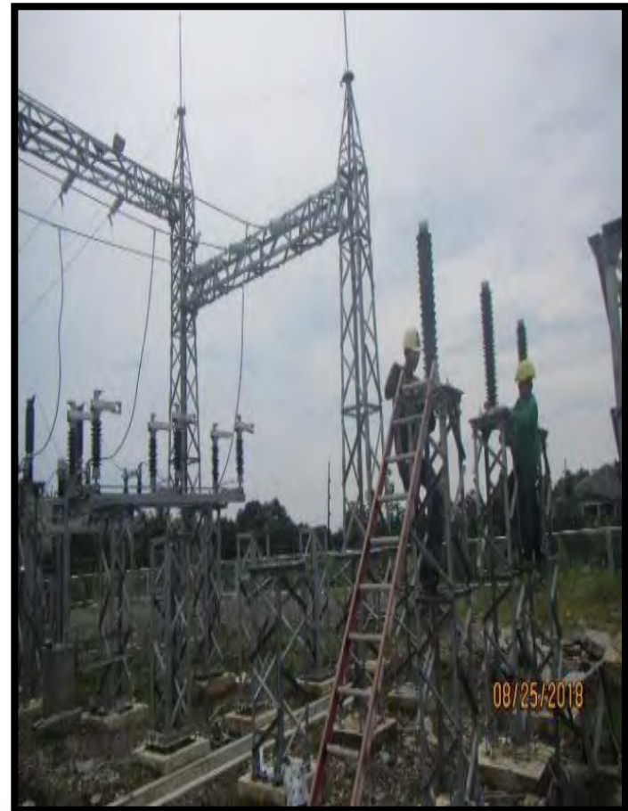
Installation of Surge Arrester
