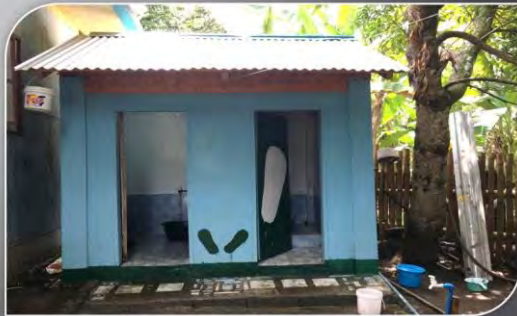
Project Title: Construction of Two (2) Units Communal Public Toilet in Brgy. Pandiaranao, Tugaya, Lanao del Sur Project Cost: PhP 53,163.00 Fund Type: RWMHEEF Power Plant: AGUS HEPs
